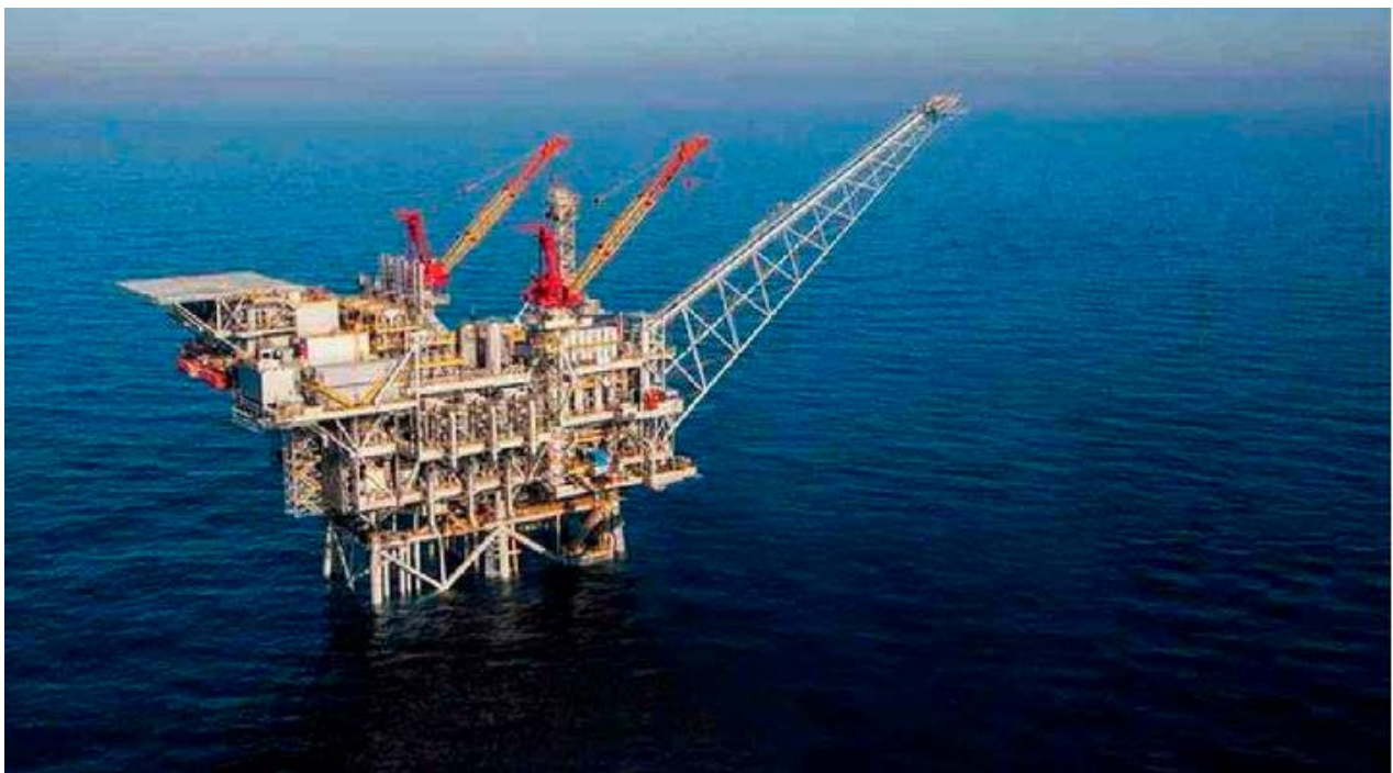
Figure 6: Bay of Bengal offshore platform
